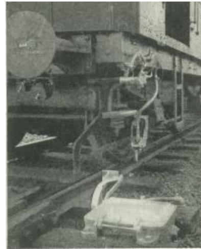
Figure 1: Trainstop and tripcock, Melbourne 1919
